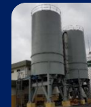
Sludge Storage Silo
